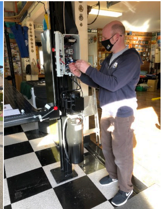
Connection to 220V by AJ's Electrical
