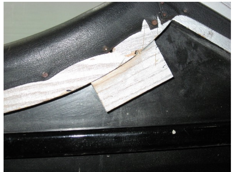
4. Door frame that has been drilled for the T-nut.
