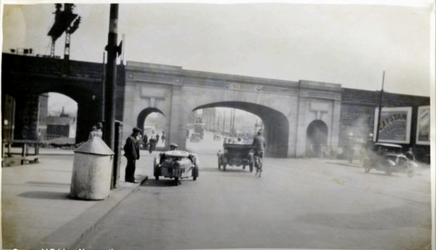
King George V Bridge, Newcastle
