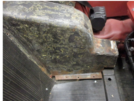
Welded but not covered
